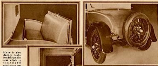
This left-rear view shows the graceful lines and ruggedness of the new Ford Sport Coupe. Strong full-crown fenders are made of 22-gauge steel.
