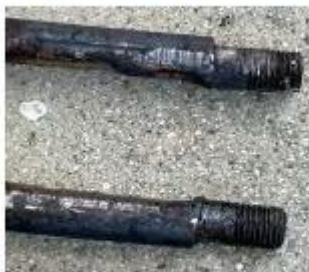
Close up of worn shackle.
