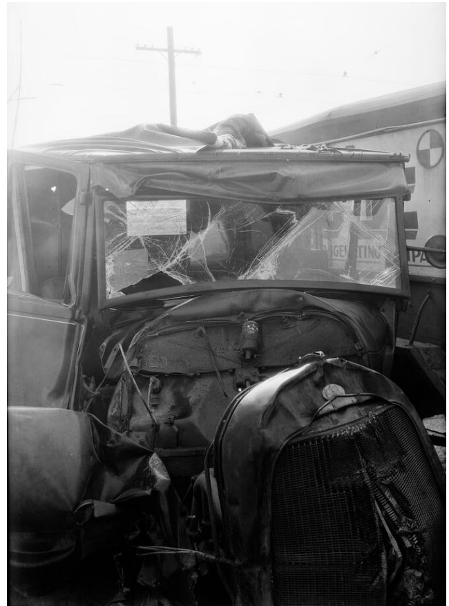
Windshield glass stayed mostly intact after the impact
