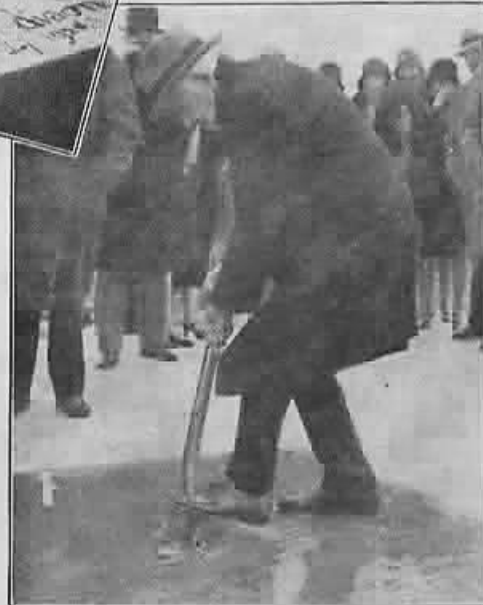
Thrusting into the wet concrete block the original spade used by Luther Burbank in his plant experiments in California.
